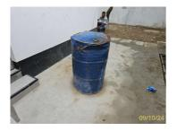
Diesel drum kept without secondary containment and label.JPEG
